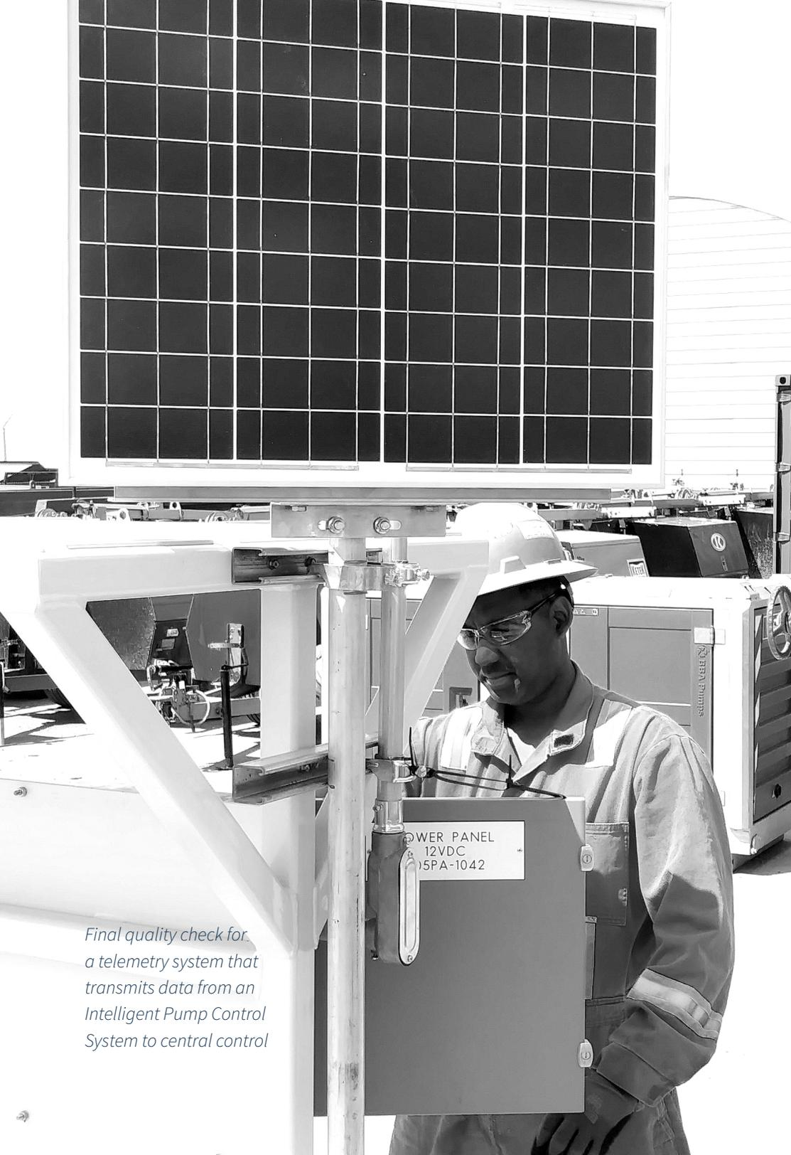
*Final quality check for a telemetry system that transmits data from an Intelligent Pump Control System to central control*
